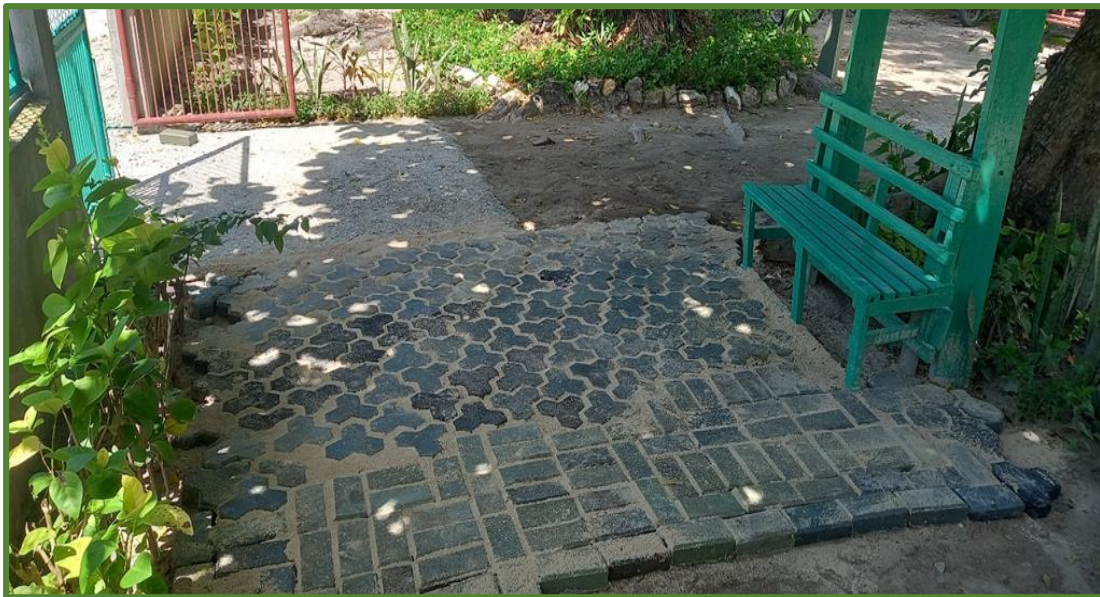
Fully cured tiles after 6 months
