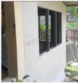
Side view of the Livelihood Facility Extension
