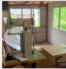
Inside of the extension to fit 3 machines inside
