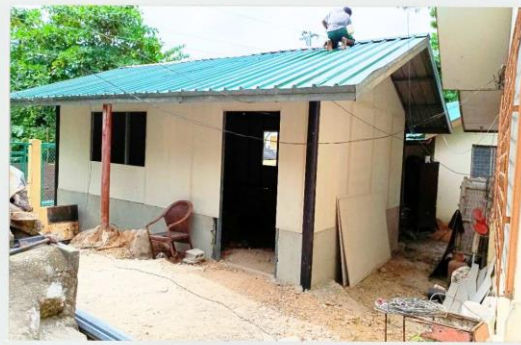
New Storage Facility (facade)
