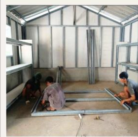
New Storage Facility (inside view)
